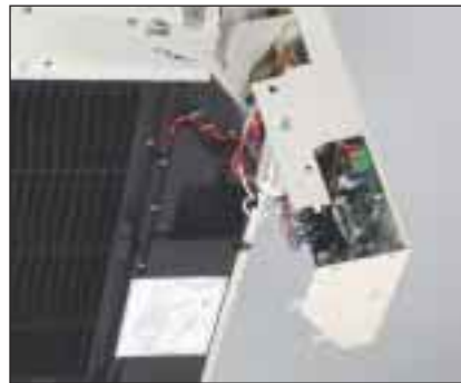
Sliding, drawer mounted electrical box. Access to all electrical connections.
